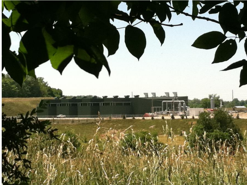
A compressor station in Washington County, PA
