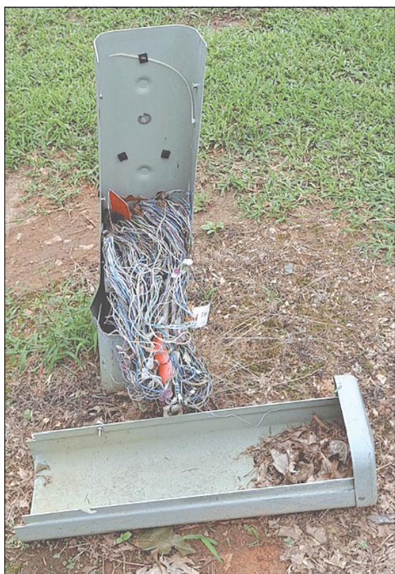
Area residents and business owners are reporting telephone and internet outages in Prince Edward and Buckingham Counties. Above are just two of the many telephone pedestals spotted in Buckingham with loose or broken covers and wires exposed to the elements.
