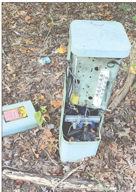
Area residents and business owners are reporting telephone and internet outages in Prince Edward and Buckingham Counties. Above are just two of the many telephone pedestals spotted in Buckingham with loose or broken covers and wires exposed to the elements.
